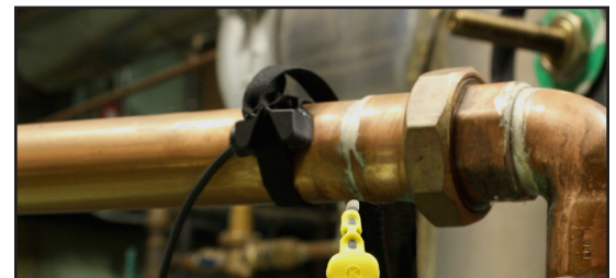
54011-K Pipe Strap Probe attached to a pipe surface.
