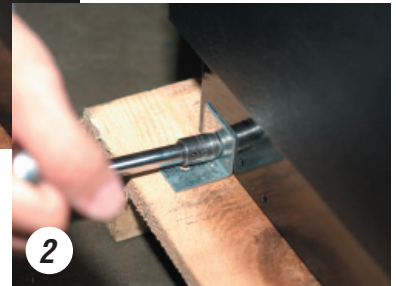
2 Removing bracket from cabinet.
