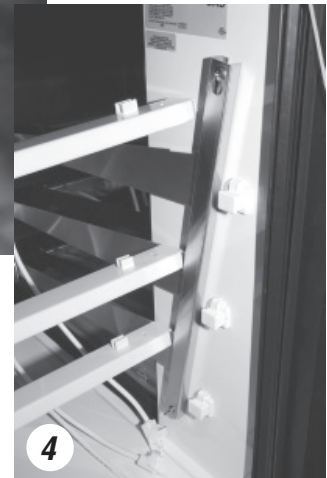
4 Install rear brackets.
