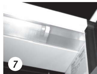
7 Interior top light assembly properly installed.
